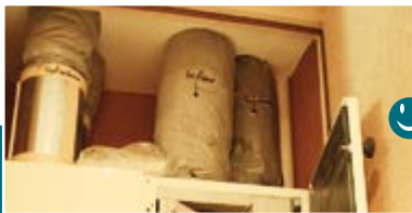
Ventilation double-flux
